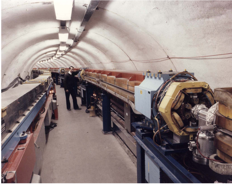
FIGURE 2. Photograph taken in the accelerator tunnel, with the synchrotron on the left and CESR on the right.
