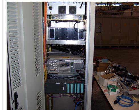
The PLC/LLRF interface is handled by a remote I/O rack, connected via Profibus communication processors (CP) to a CPU in the cavity control rack on the storage ring.
