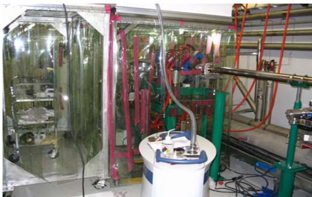
Portable cleanroom for beam pipe attachments in the tunnel
