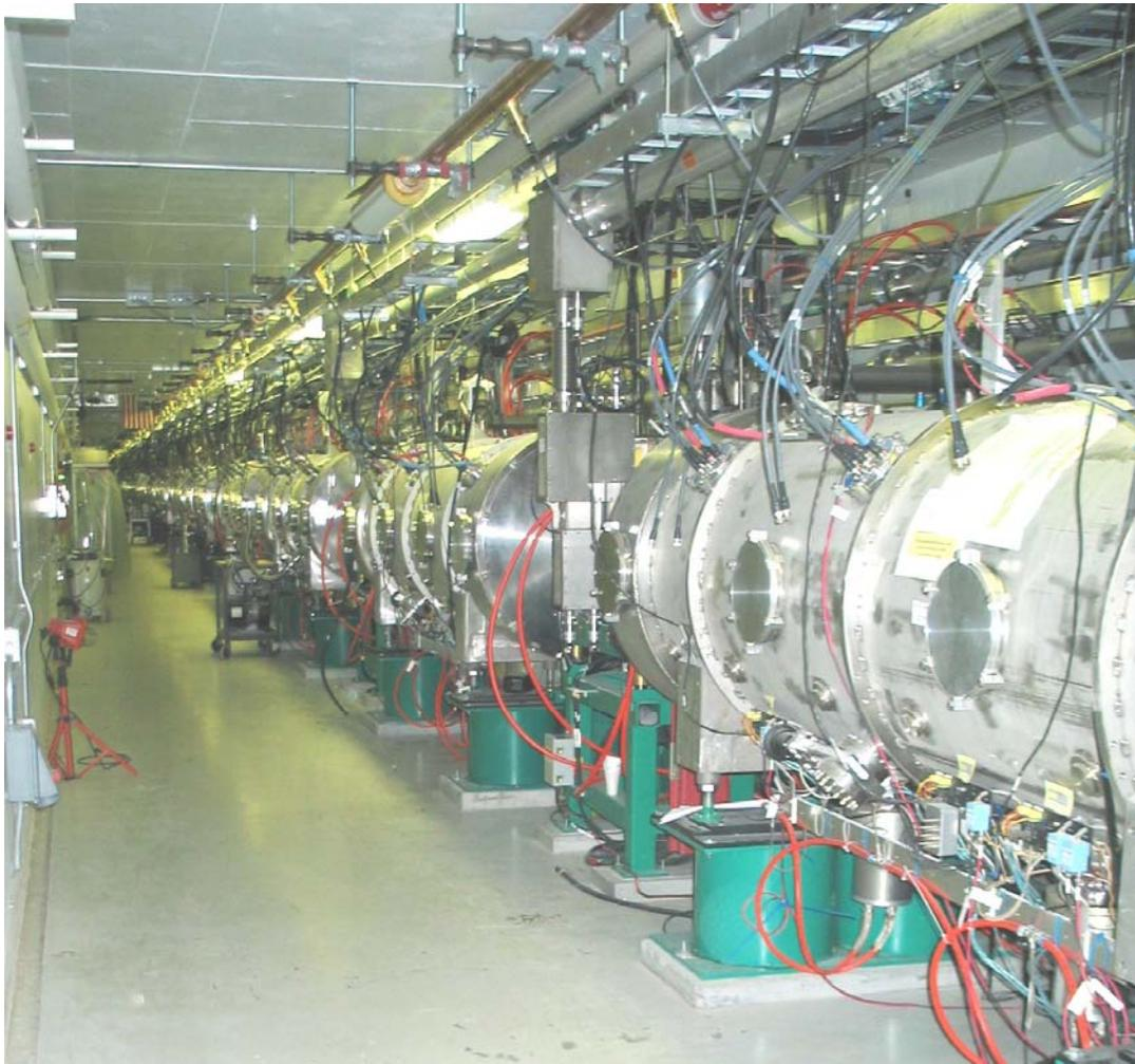
Performed microphonics and seismic measurements at 4.2 K on selected cavities with JLab and MSU
