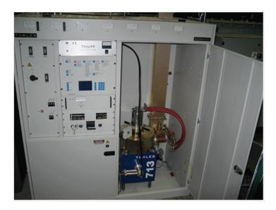
Figure 4.4.3: IOT inside the transmitter.
