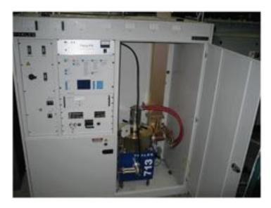
Figure 4.4.3: IOT inside the transmitter.
