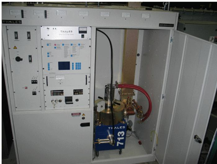
Figure 2.3.15: IOT inside the transmitter.
