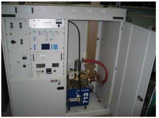
Figure 3: TH 713 IOT inside the transmitter.
