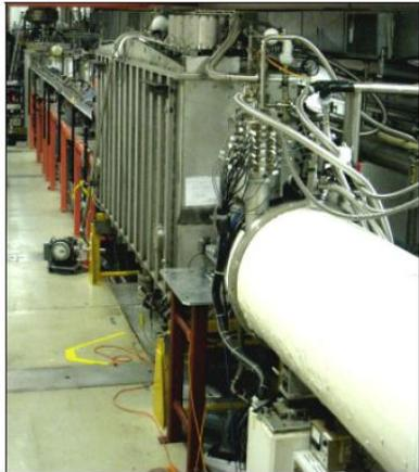
Energy upgrade cryomodule in the ATLAS tunnel.
