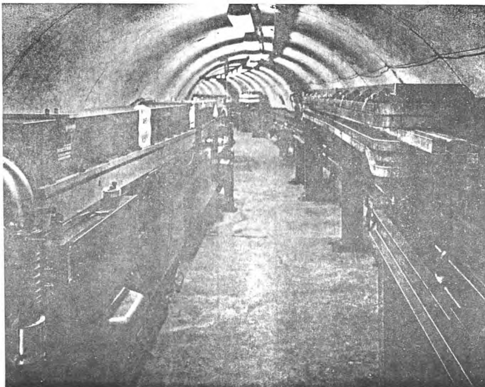
Fig. 1-2 Synchrotron tunnel with a prototype of storage ring dipole magnet in place.
