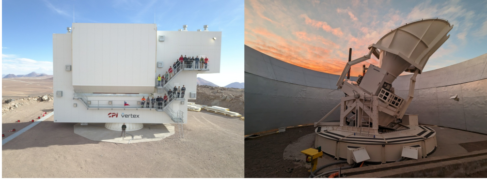
Figure 1.5: Left: The Simons Observatory Large Aperture Telescope after installation on Cerro Toco. Many members of SO are shown for scale. Photo credit: Rolando Dunner. Right: One of the SO Small Aperture Telescopes inside its ground screen. The main structure that is visible is the forebaffle that blocks out stray light; the SAT itself is located in the center of the structure mounted above the center of the platform. Photo credit: Nicholas Galitzki.
